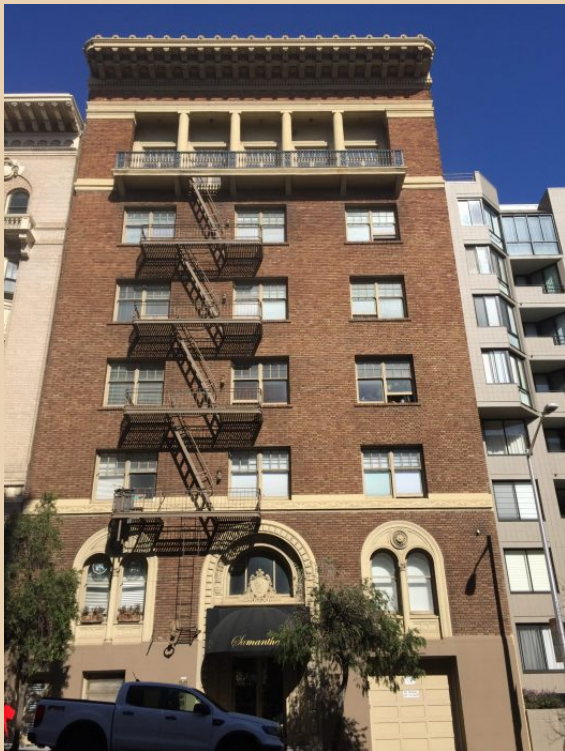
The Samantha apartment building.
